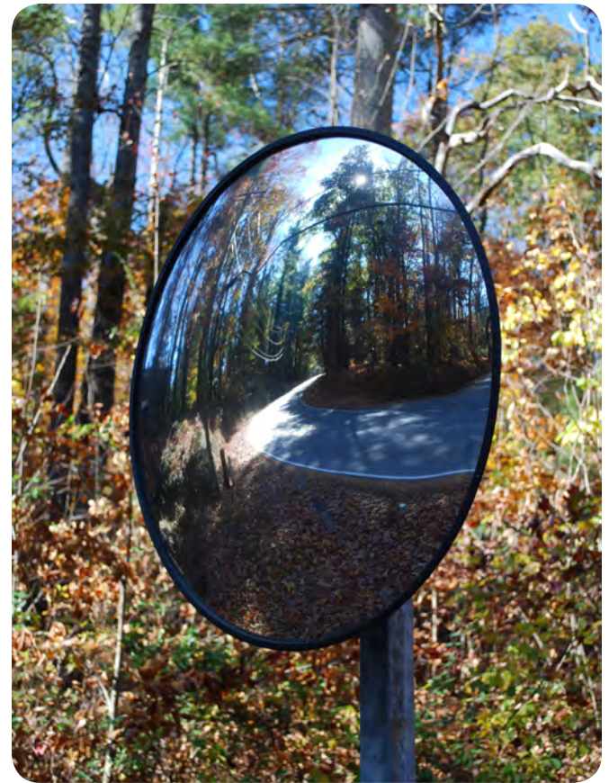
Convex mirror provided to allow motorists to see around the curve
