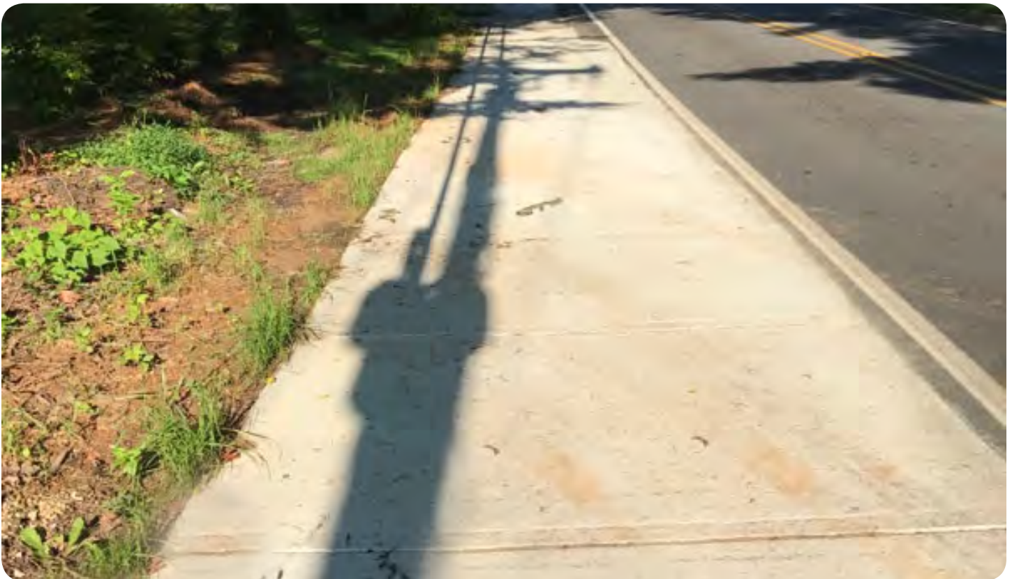
Existing Laurel Park Highway Sidewalks
